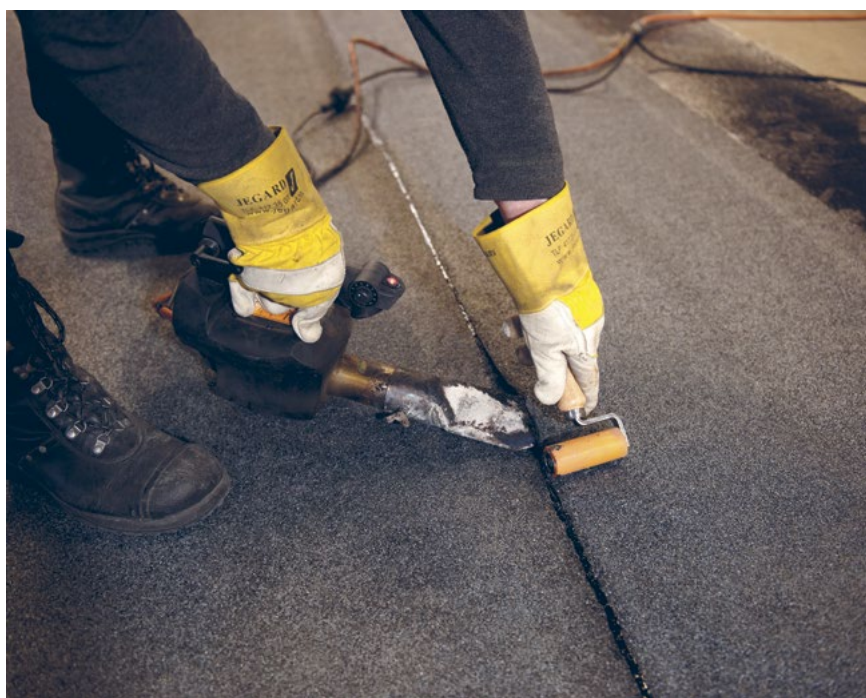
■ A hand-held hot air welder, for use in roofing operations, is an example of a burner with shielded combustion.
